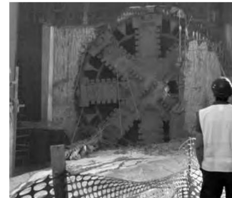
TBM passes directly through the GFRP soft eye diaphragm wall
