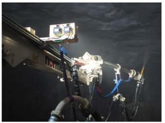
TamShot 110AF is used for wet mix sprayed concrete processes in the tunnelling and mining industry. The product is applied where initial ground support is needed or where a permanent lining has been designed (such as for single shell tunnel lining).
