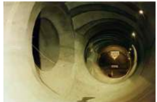
CombiShell™, Heathrow Baggage Tunnel, London, UK
