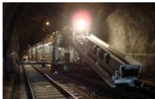
Equipment for rail tracks dismantling, Arlberg Tunnel – Safety Engineering Upgrade, Langen, Austria
