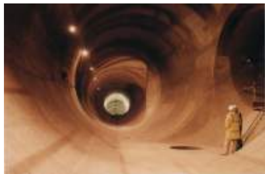
CombiShell™, Heathrow Baggage Tunnel, London, UK
