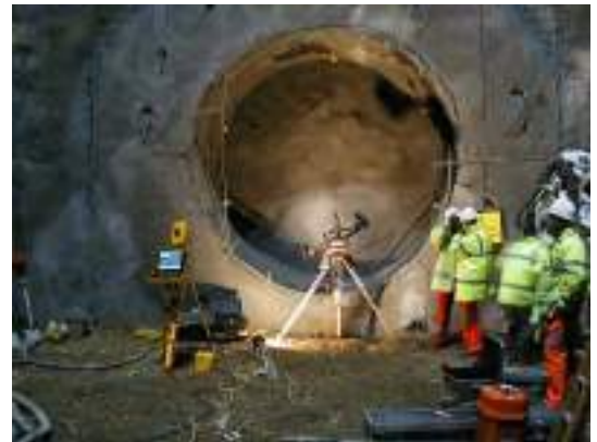
Tunnelbeamer™ and LaserShell™, Heathrow Terminal 5, London, UK
