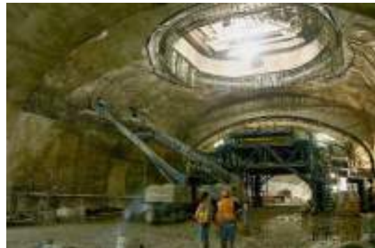
Weehawken Tunnel and Bergenline Avenue Station, Weehawken, New Jersey, USA
