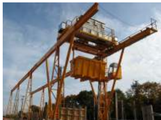
Muck shaft-hoist, Lainzer Tunnel LT 31, Vienna, Austria
