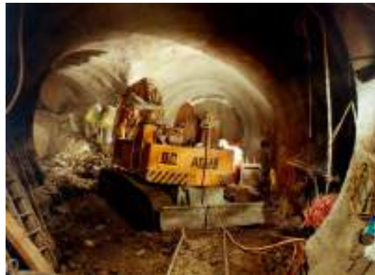
CombiShell™, Heathrow Baggage Tunnel, London, UK
