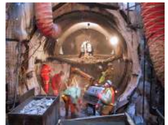
NATM in frozen ground, UWWTD Flow Transfer Works, T3 Tunnel Recovery Program, Hull, UK
