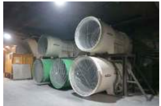
Main Ventilation Plant Arlbergtunnel - St. Anton, Austria
