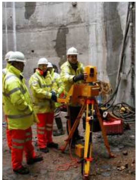
TunnelBeamer™ Training, Heathrow Terminal 5, London, UK
