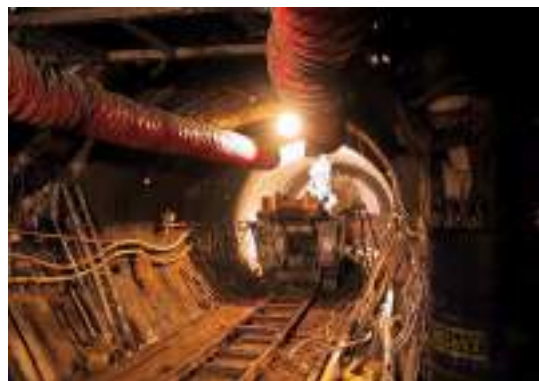
UWWTD Flow Transfer Works, T3 Tunnel Recovery Program, Hull, UK
