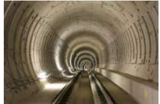
Metro TBM, Razeny, Czech Republic
