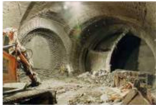
CombiShell™, Heathrow Baggage Tunnel, London, UK
