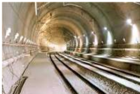
North Downs Tunnel, Rochester, UK
