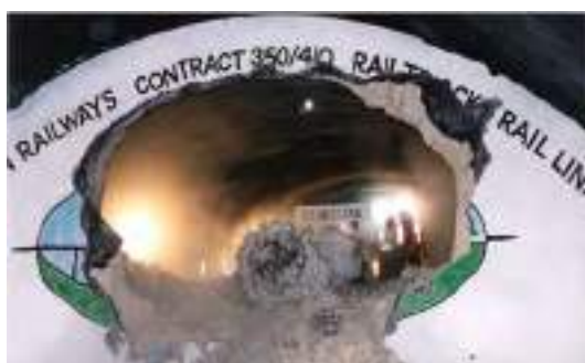
North Downs Tunnel, Rochester, UK
