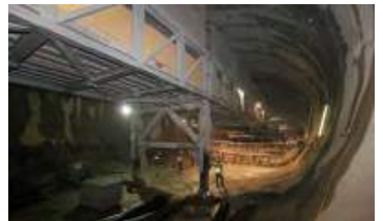
Achrain Tunnel, Dornbirn, Austria
