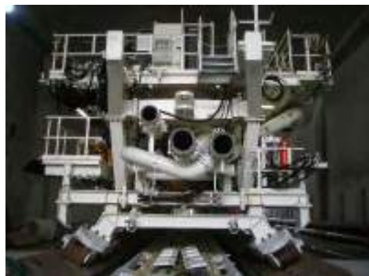
Backup Slurry TBM, Metro Karlsruhe, Germany
