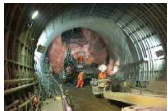
LaserShell™ with SGI-Lining, Kings Cross Station Redevelopment, London, UK
