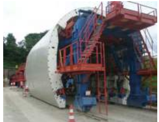
Vault shutter/formwork , Schluechterner Tunnel, Schluechtern, Germany
