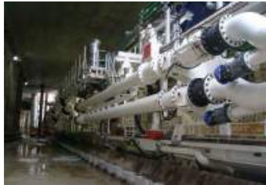
Backup Slurry TBM, Metro Karlsruhe, Germany
