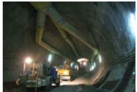
Ventilation system side wall drift, Lainzer Tunnel LT 31, Vienna, Austria
