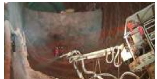
TunnelBeamer™, North Downs Tunnel, Rochester, UK
