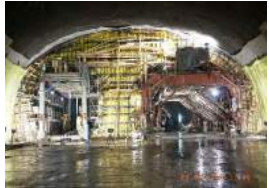
Blisadona Tunnel, Arlberg, Austria
